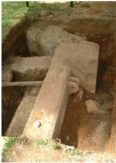
Figure 9. Drawbridge Superstructure (FTK 31, 32, 38 and 39).
