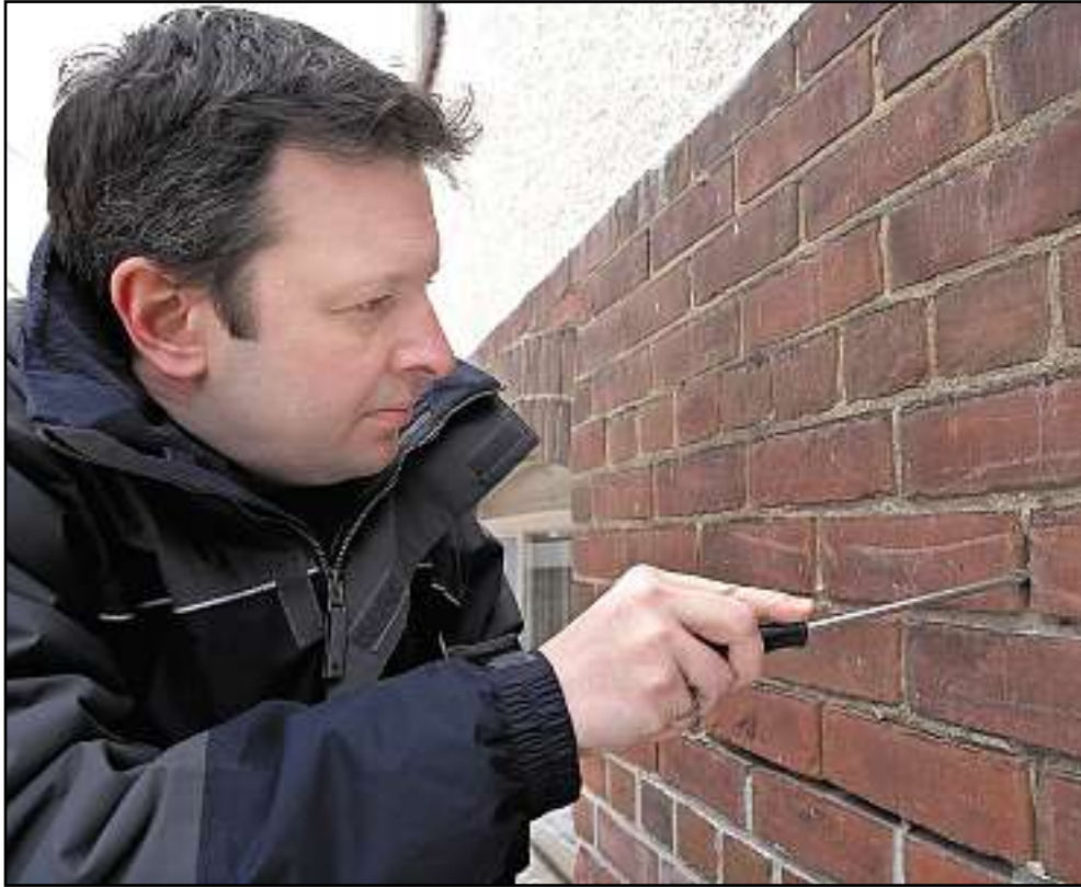
Seneca instructor Graham Clarke examines the exterior of a home, checking for loose mortar. Clarke also works for Carson Dunlop and Associates, the company that delivers the Home Inspection program in partnership with Seneca.
