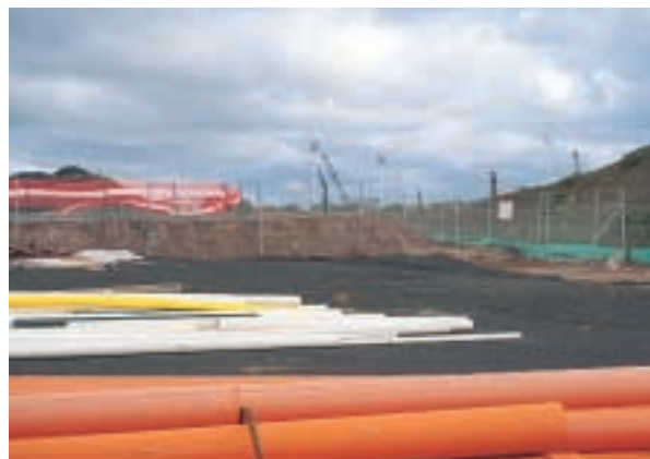
PVC pipes at the Olympic site, January 1997
