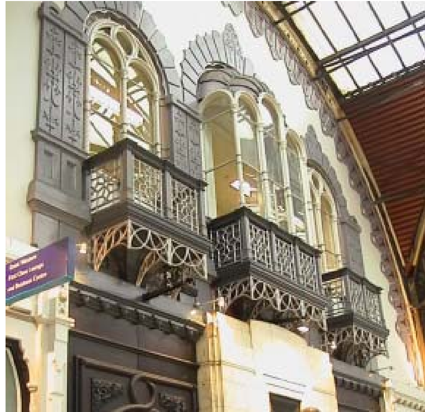
Platform 1 – Oriel windows
