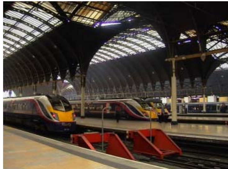
Paddington station general view of main area
