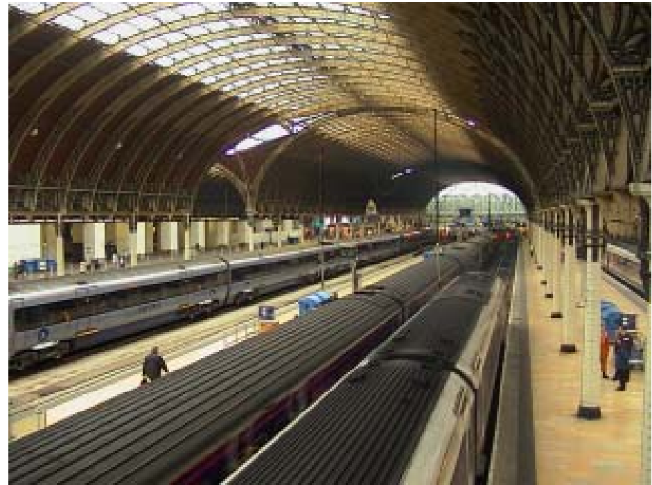
Central roof span
