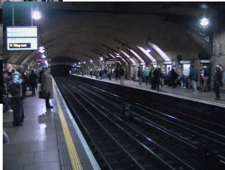
Crossrail – Paddington Station
