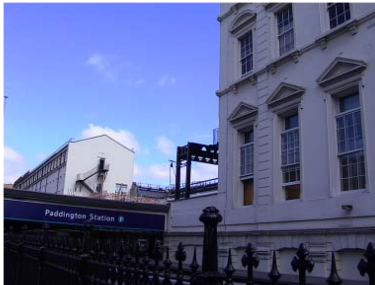
The 'gap' in the buildings
