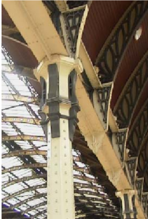
The steel columns and iron ribs and girders
