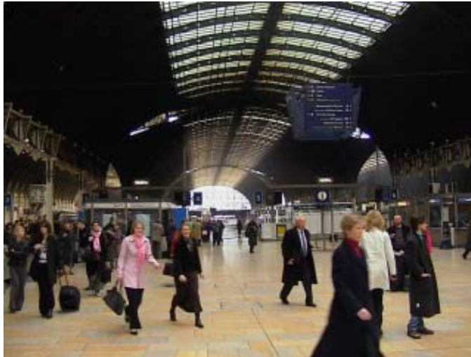
Paddington station general view of main area
