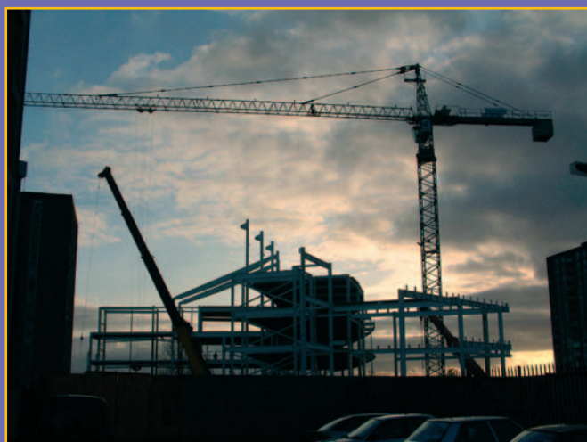
Civic Centre under construction by Bennett Construction
