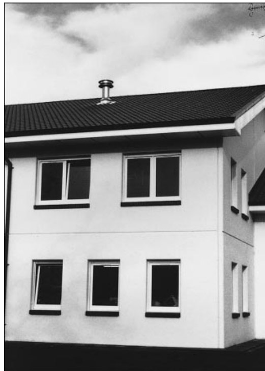
Fig. 10. Painted finish, Watchtower offices, Co. Wicklow, Ireland
