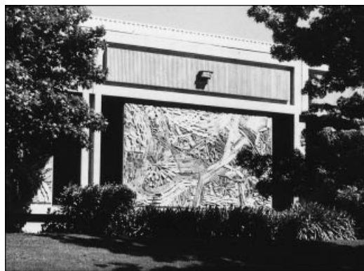
Fig. 9. Hand-laid rock finish, Sacramento, California
