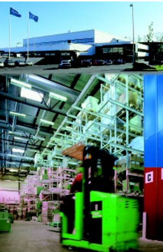
Office building of LVI-Dahl Oy, Vantaa.
