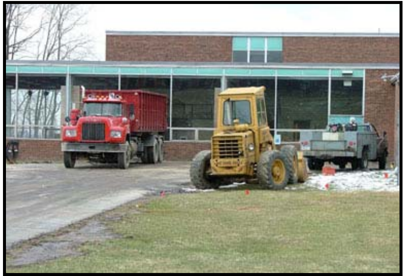
Demolition begins on the Middle School renovation project.— March 2004
