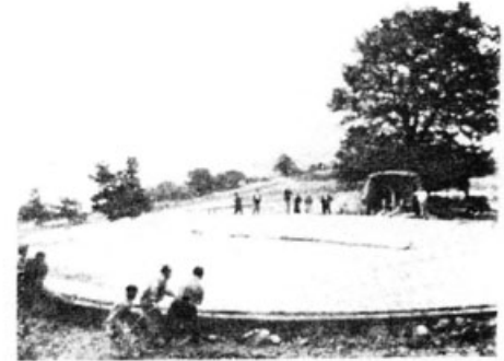
Fig. 5 Laying of the external membrane.
