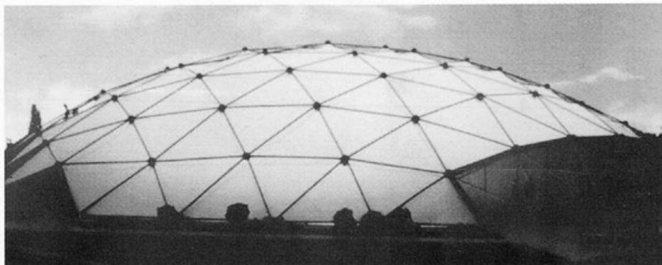
Interlocking pipes covering a polyester membrane are raised with air in an hour.
