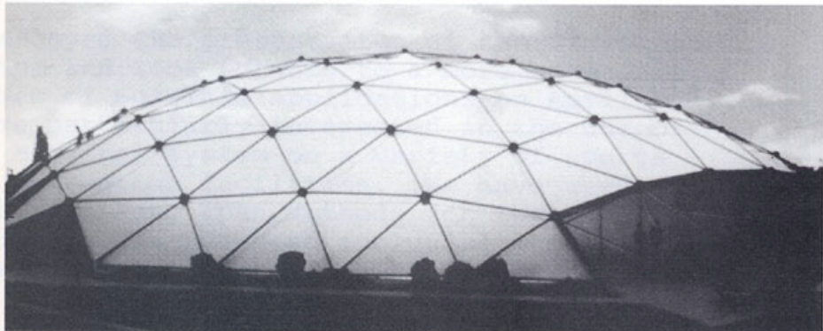
Interlocking pipes covering a polyester membrane are raised with air in an hour.
