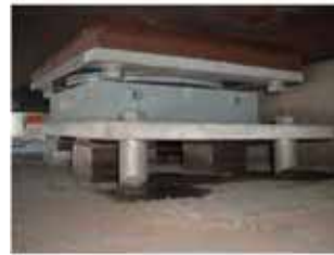
Finally resting on Pot Bearings
