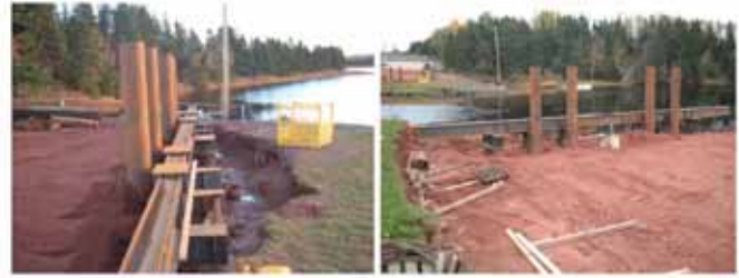
Temporary Abutment Construction
