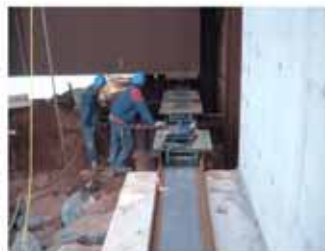
Placing Hillman® Rollers
