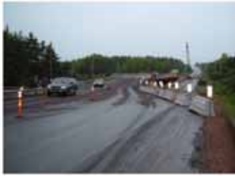
Traffic Re-routed onto Bridge
