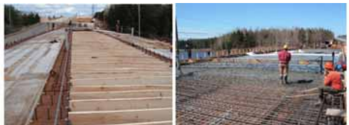
Forming for new Concrete Deck
