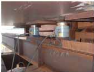
Jacking Bridge Up
