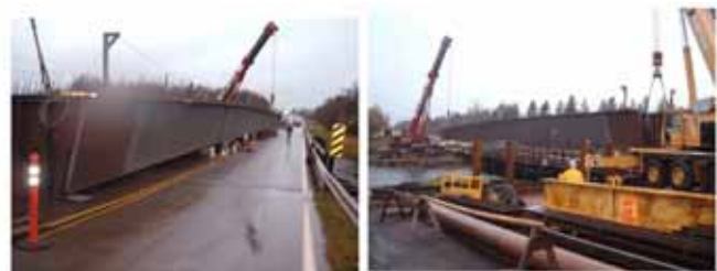
Erecting girder on existing bridge
