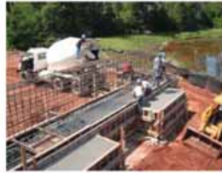
Placing Concrete Abutments
