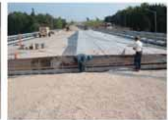
Applying Waterproofing Membrane
