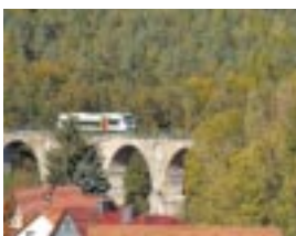
Regio-Shuttle am Viadukt in Sonneberg West
