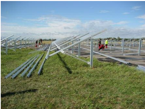
Mounting of the structure to carry the modules
