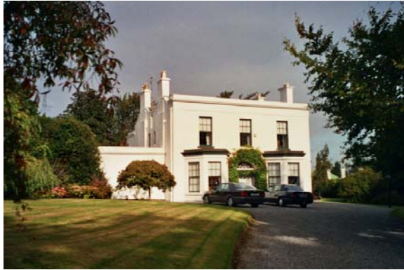
Fig. 9 Hillside, which dates to the mid 19 th century
