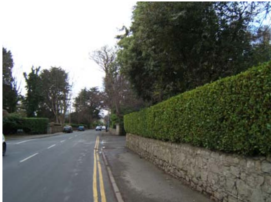
Fig. 7 View of roadside boundary
