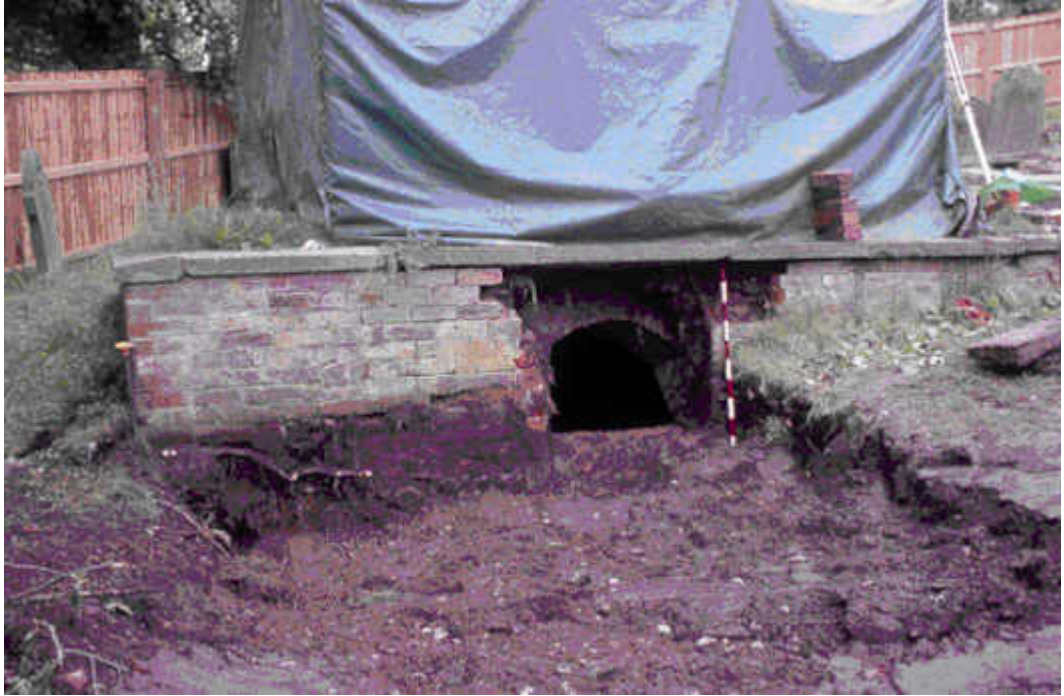
Plate 7: Vault 213, north-east facing
