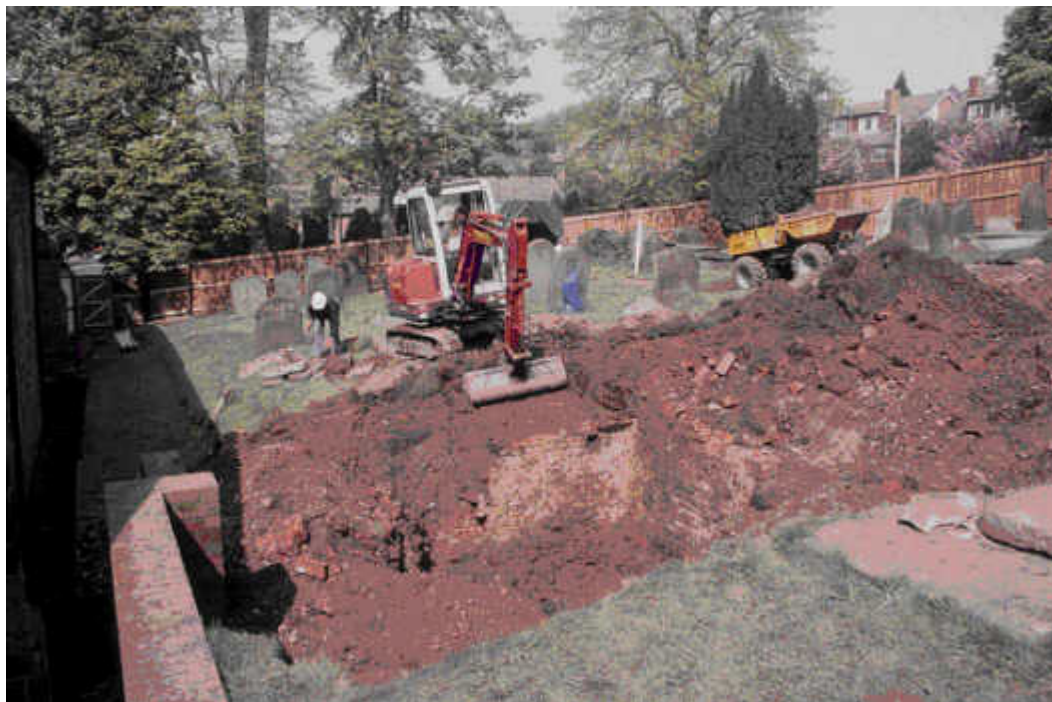
Plate 3: working shot, vicinity of vault 3
