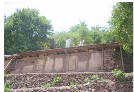
Fig 25: Traditional timber and stone house is undamaged, Ghanool, Balakot.
