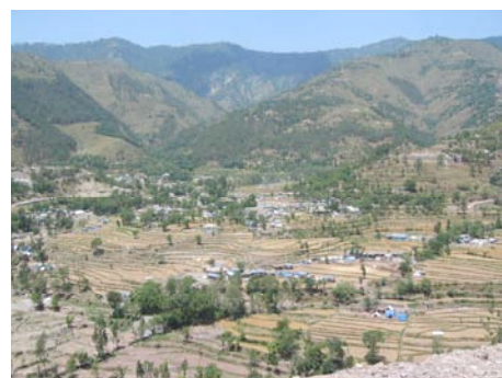
Fig 32: Terraces plowed and awaiting replanting, Balakot.
