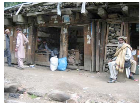
Fig 26: Road side shop of traditional construction undamaged, Jared, Kaghan Valley.
