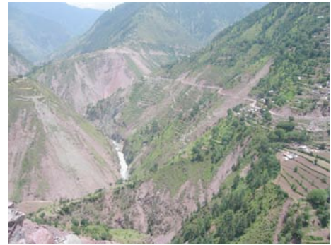
Fig 13: Landslides on the main Kaghan Valley road.
