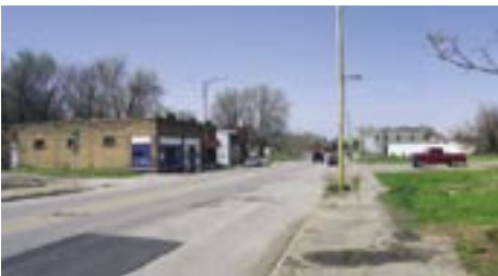
Existing 24th Street Corridor
