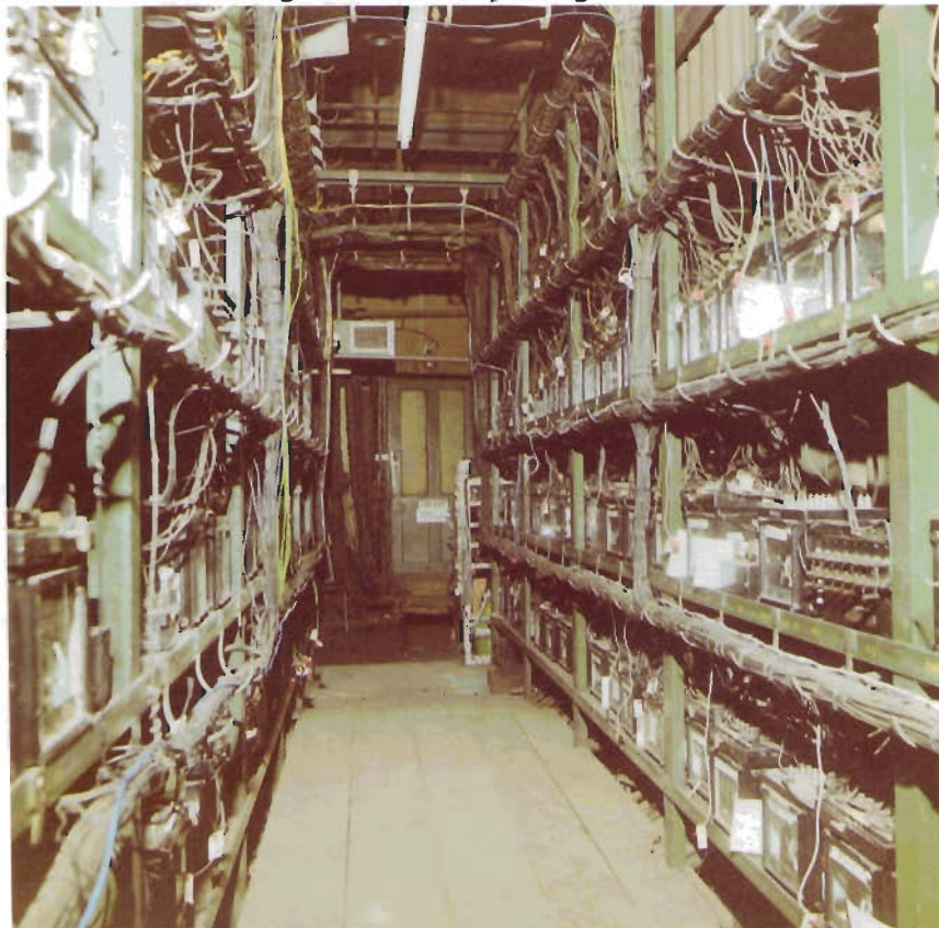
Fig 11. A view of the relay room, looking towards the entrance, showing the relay racks, and the trees of the wiring. Relays TRR DM and TRR DN are on the bottom shelf on the right in the last section towards the door.
