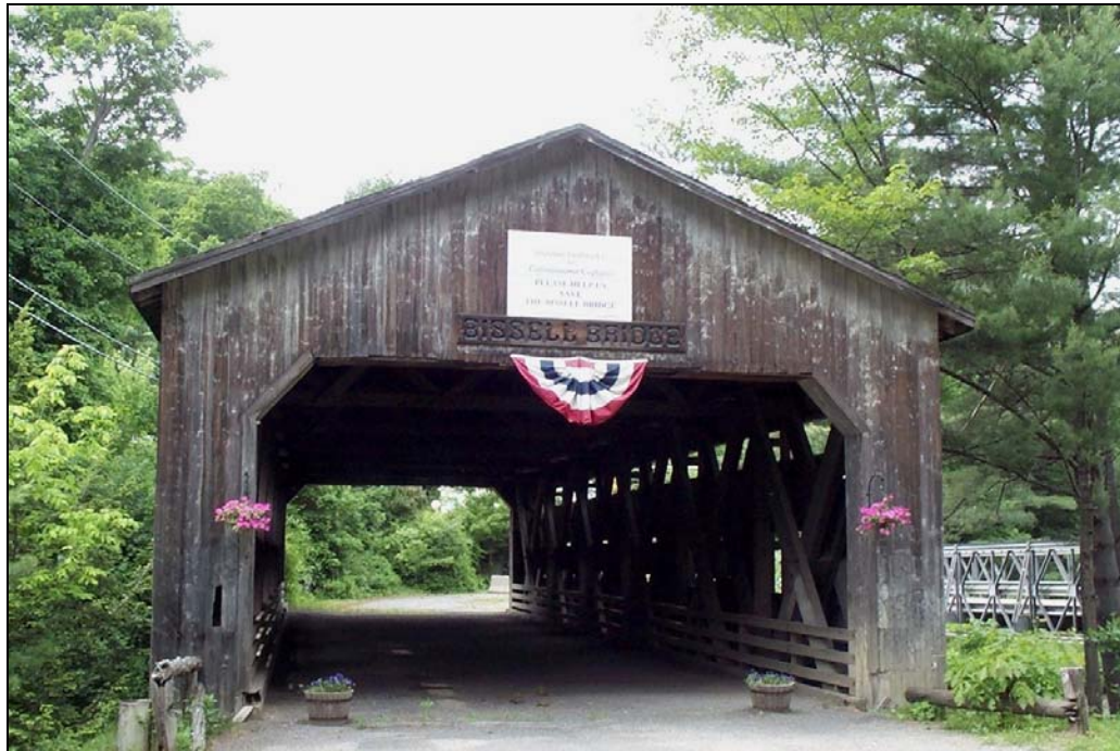
Bissell Bridge is one of a number of covered bridges in Franklin County
