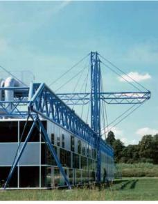
The concept for INMOS is large, column-free flexible and universally serviced open operational spaces with a central circulation spine and central meeting space at its heart.
