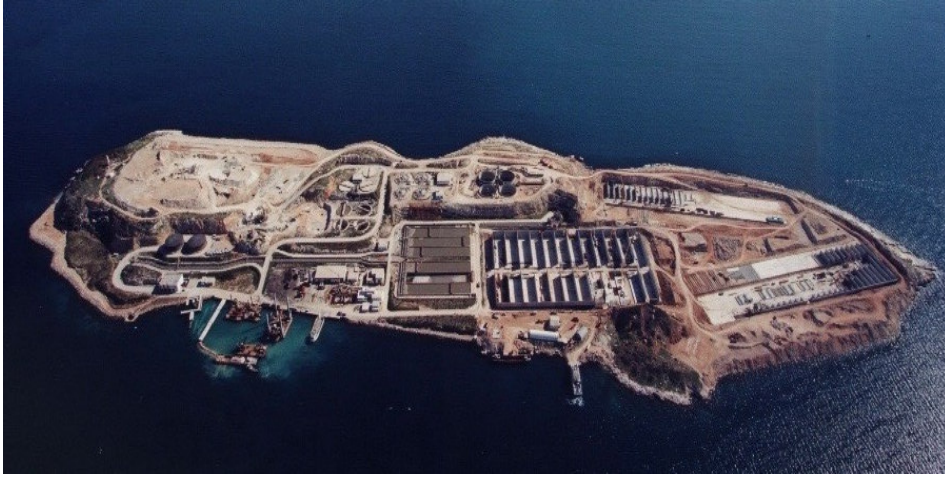
Wastewater Treatment Plant of Psytalia
