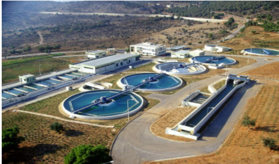
Water Treatment Plant of Aspropyrgos
