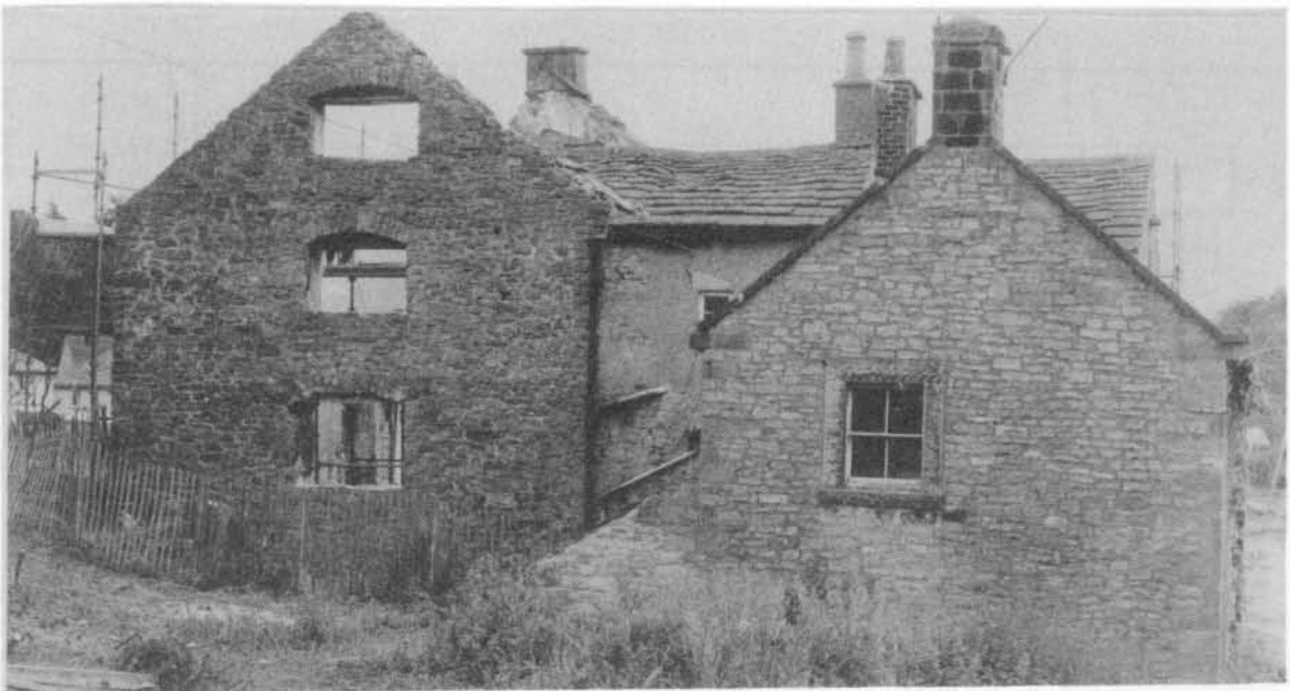
Calver Mill - the mill building is on the left, with the wheelpit protected by the chestnut paling. The centre building is later, linking the mill to the possibly older building, right.
