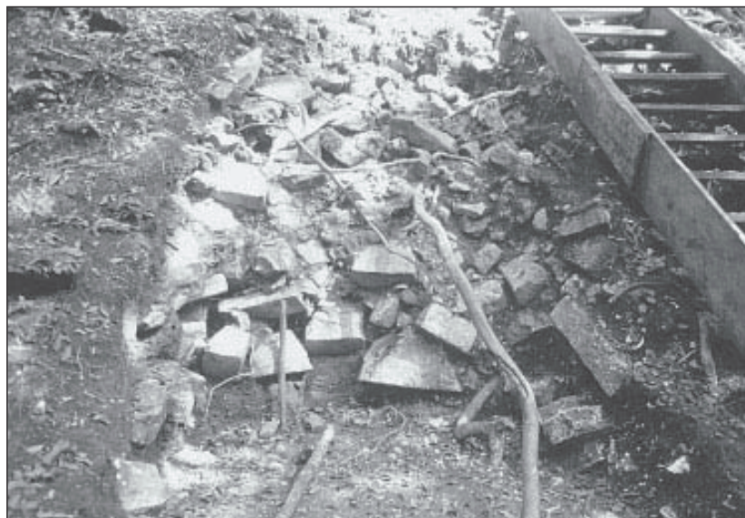
Figure 4 Faced wall during excavation. Note the presence of soil and mortar used in backing masonry as well as collapsed cut stones.
