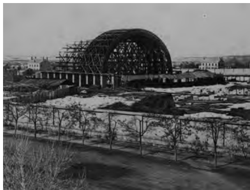
Construction of the Salt Lake Tabernacle
