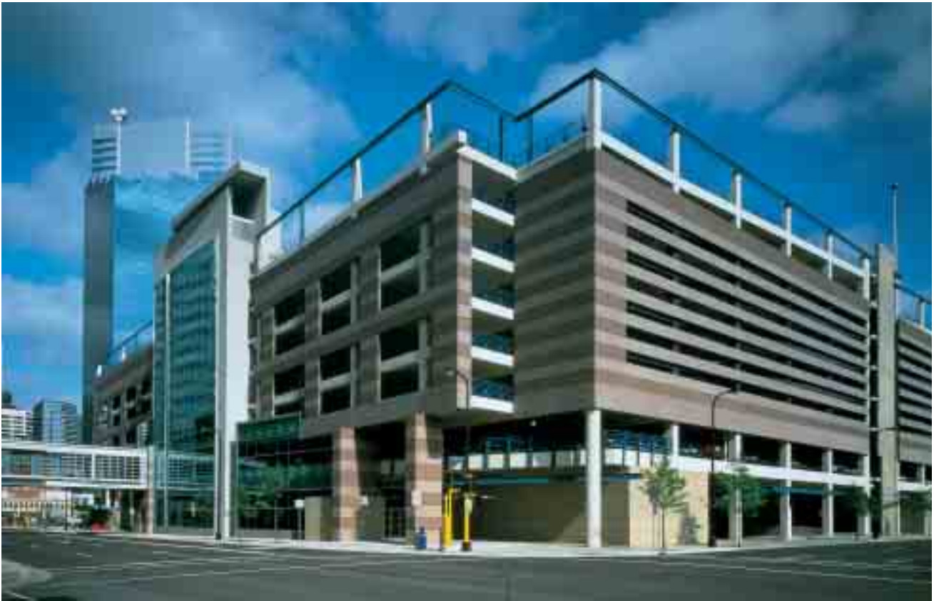
Located in the Convention Center District of downtown Minneapolis, the Leamington Municipal Transit Hub relates in material and color to the nearby Convention Center. The architects decided to use precast cladding to express the design as a veneer instead of having the structural system dictate the design. Photo: Jon Miller/Hedrich-Blessing
