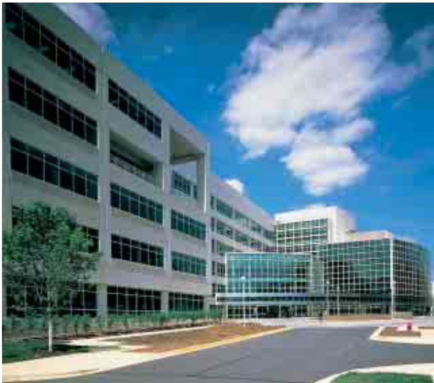
Six-inch-thick precast panels on the exterior of the National Archives & Records Administration building in College Park, Md., prevent much sunlight from penetrating the interior, where valuable records are stored. The use of precast also helps maintain the required temperature and humidity. Photo: Maxwell Mackenzie
