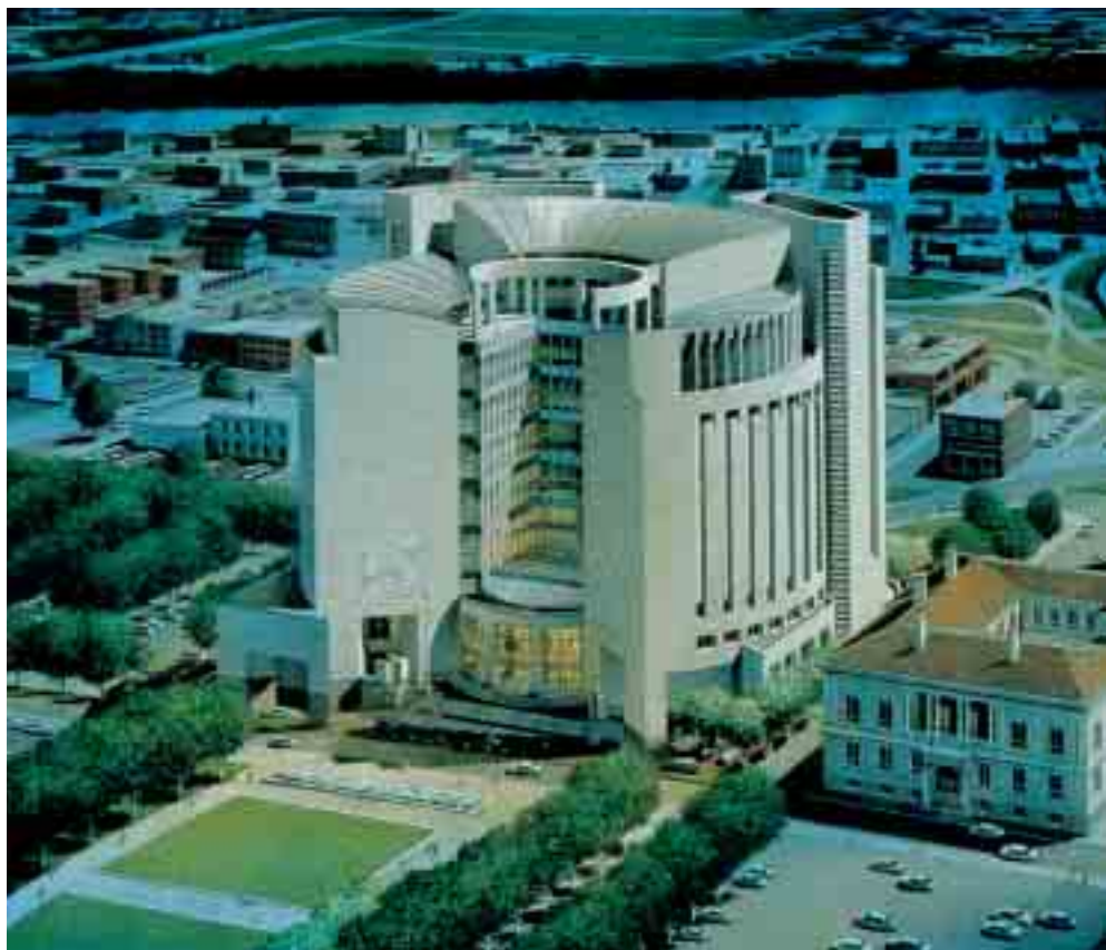
Designed in association with Abend Singleton, Associated Architects, the crescent-shaped Charles Evans Whittaker United States Courthouse in Kansas City, Mo., features curved walls, with shaped pieces of precast concrete cladding wrapped around the corners. Precast was selected for the facade because it related to surrounding limestone government buildings and adapted well to the building's complex geometry. Photo: Architectural Photographics 1994, Kansas City, Mo.
