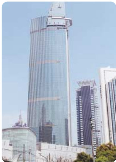
The high-rise offices of Tose Software (Shanghai) in the Fushan District
