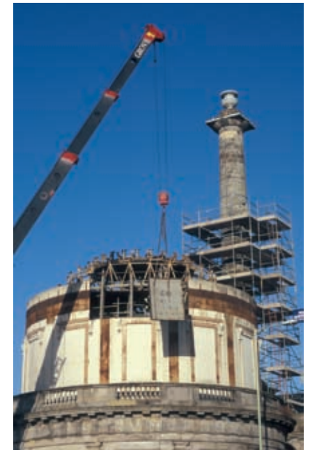
Removing the cast iron panels
