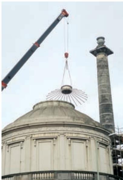
Removing the cupola
