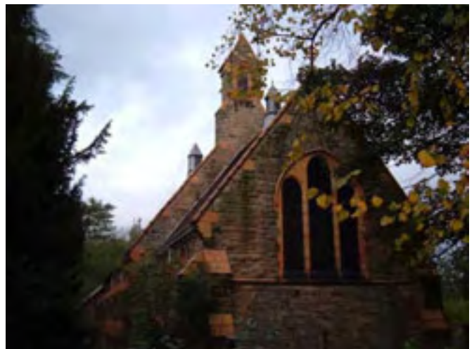
4. St. Mary's Church, built in 1901 in Early English Gothic style, adds variety and scale to the street scene.
