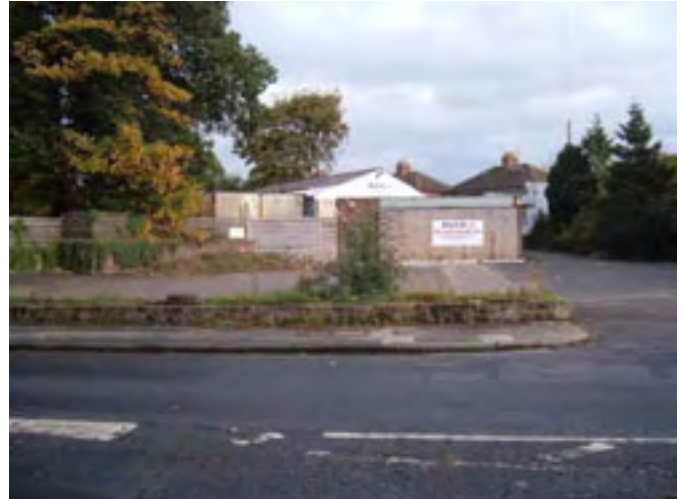
14. Vacant business premises do not present a positive image when arriving from the east.
