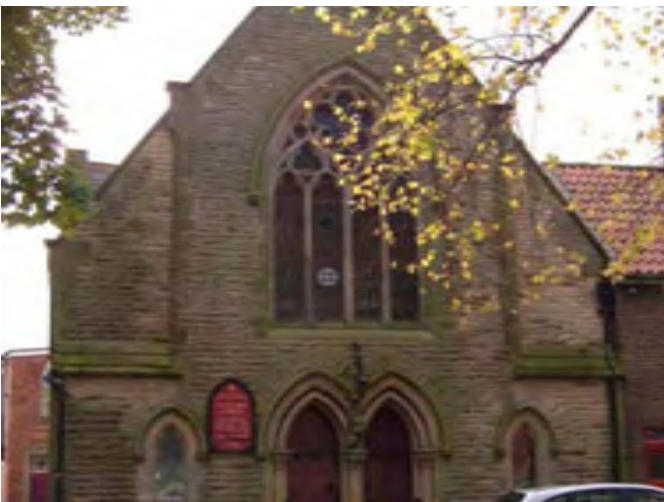
9. The 1875 Wesleyan Methodist Chapel, in 19th Century Gothic style in stone with a slate roof. Of local architectural importance.
