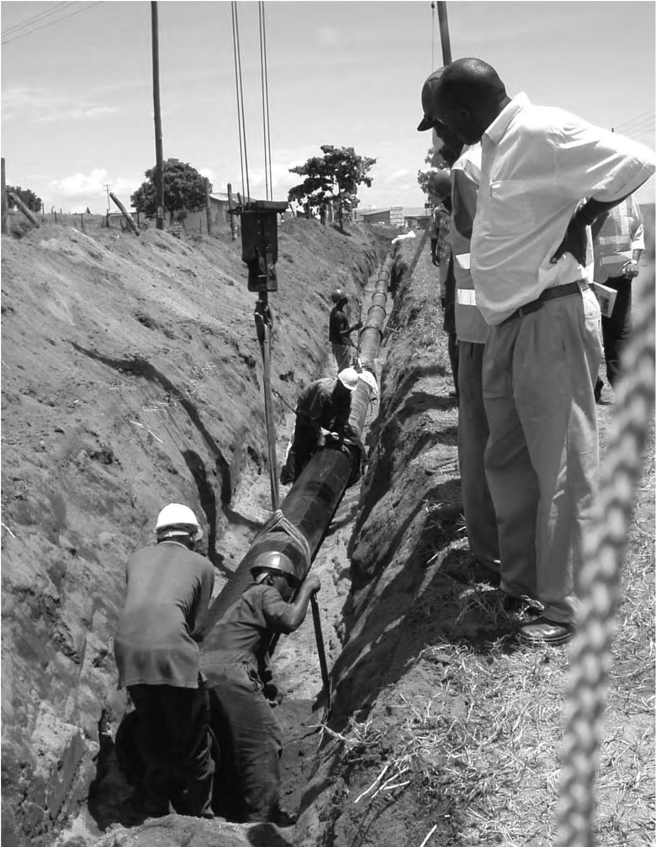
Laying of new pipes by NWSC
