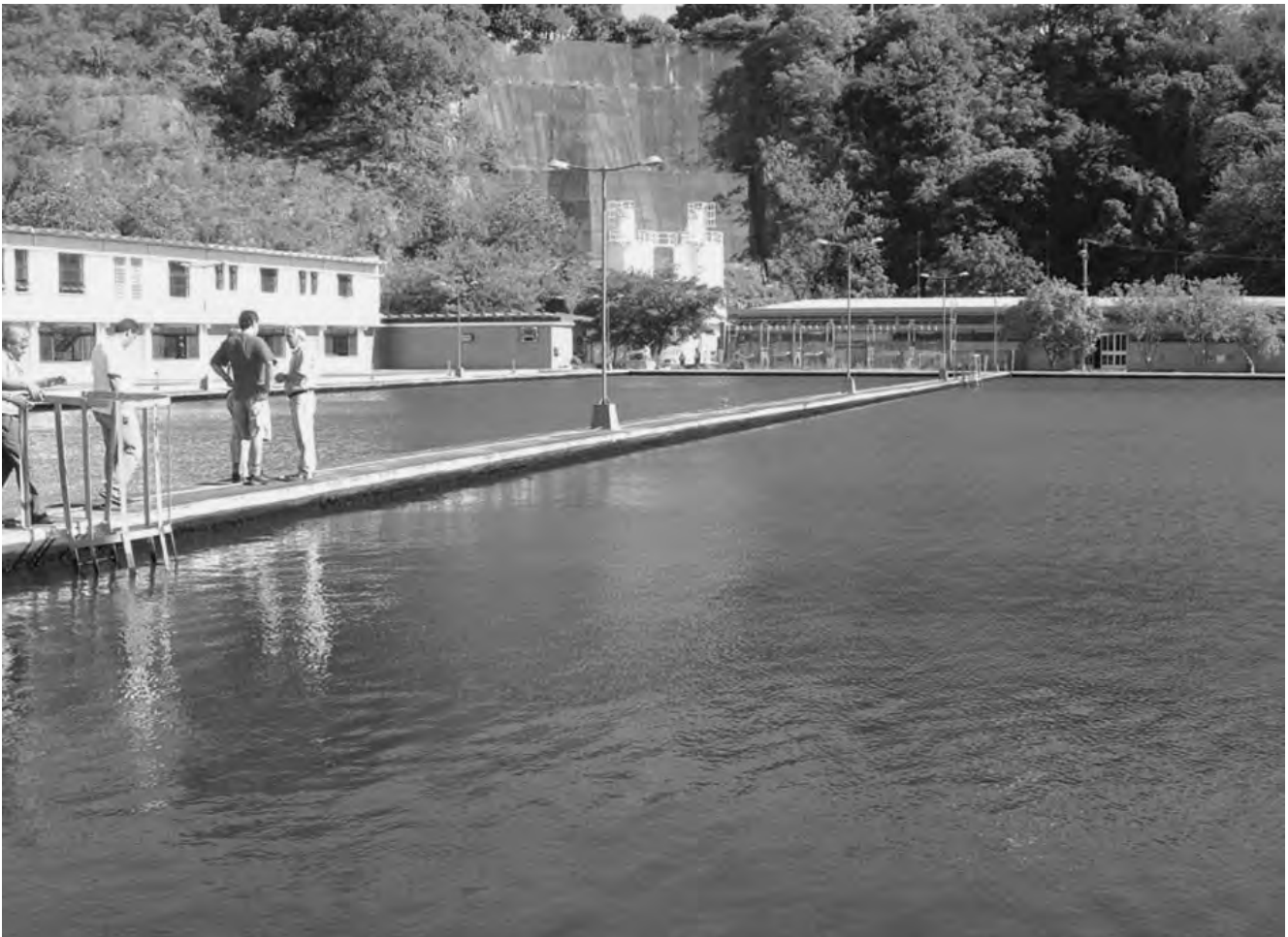
A water treatment station funded by the Porto Alegre municipality
