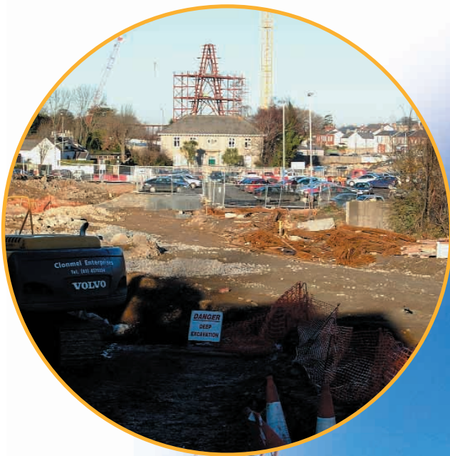
CONSTRUCTION SITE AT TANEY BRIDGE
