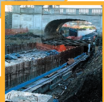
CONSTRUCTION WORK AT RIALTO
