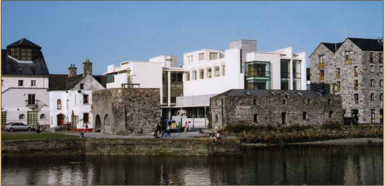
The new museum seen from the Wolfe Tone Bridge, with the old museum and the Spanish Arch in the foreground. Photograph by Ray Shanley for Galway City Council.
