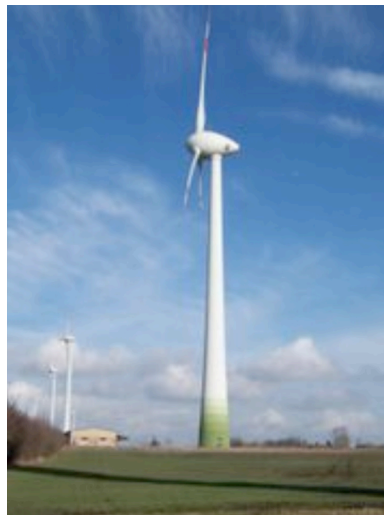
Figure 3: Enercon E-112 4.5MW turbine wind turbine located near Magdeburg, Germany.
