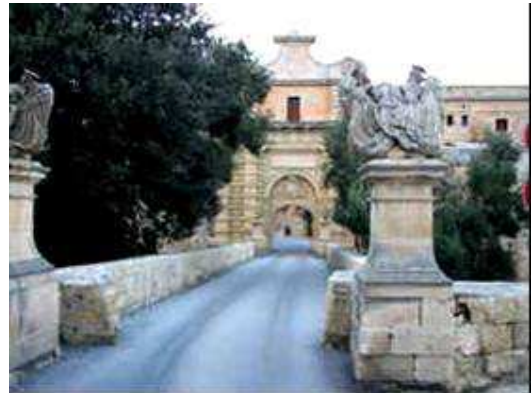
Mondion's new Mdina Main Gate
