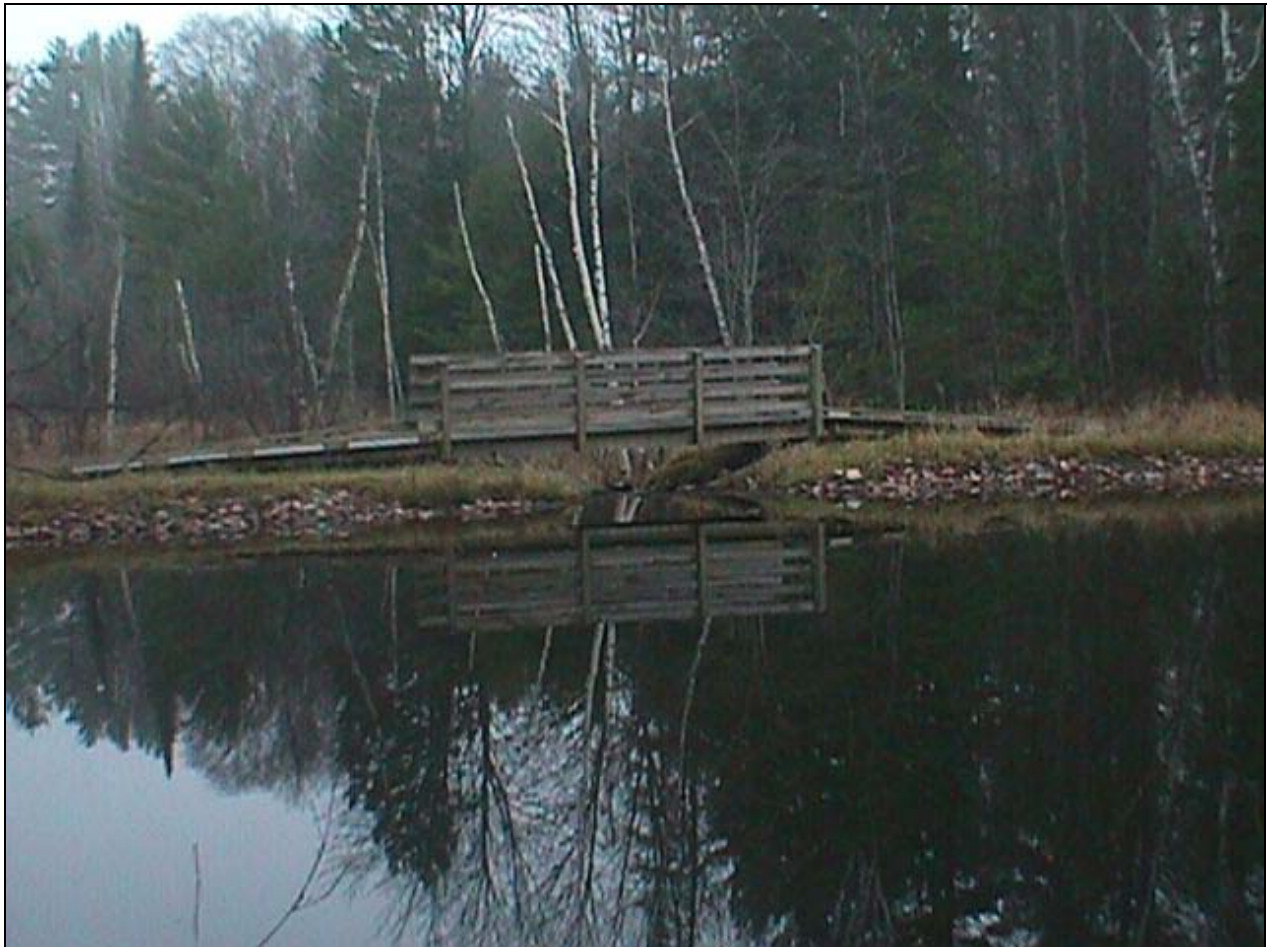
Council Lake Dam
