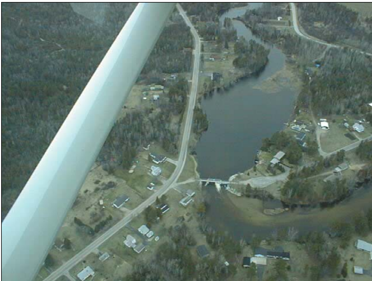
Indian Lake Dam
