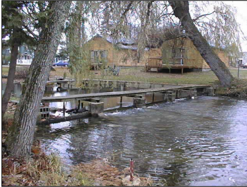
Portage Creek Dam (South Manistique Lake) at low flow with all stop boards removed.
