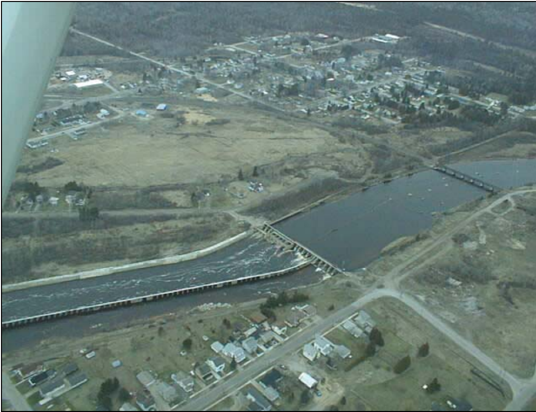
Upstream View of MPI Dam
