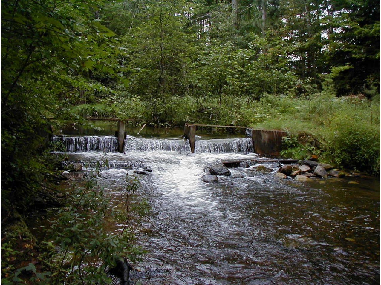
Carr Creek fish barrier dam.
