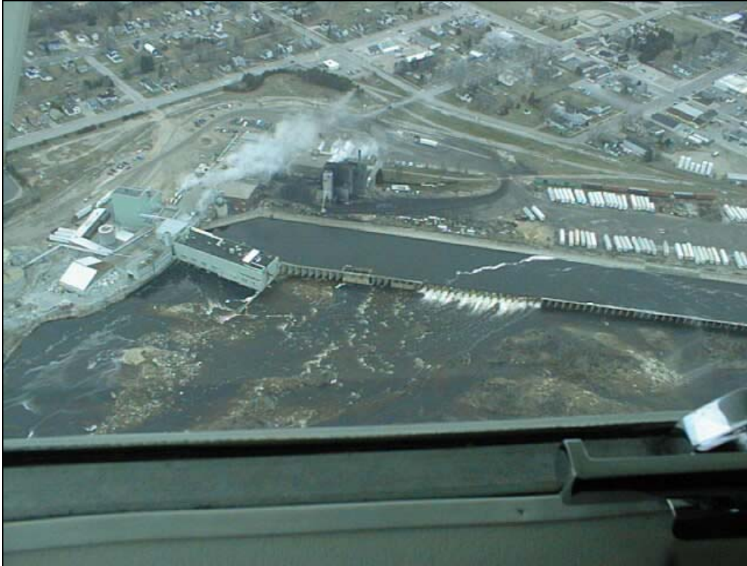
Downstream View of MPI Dam
