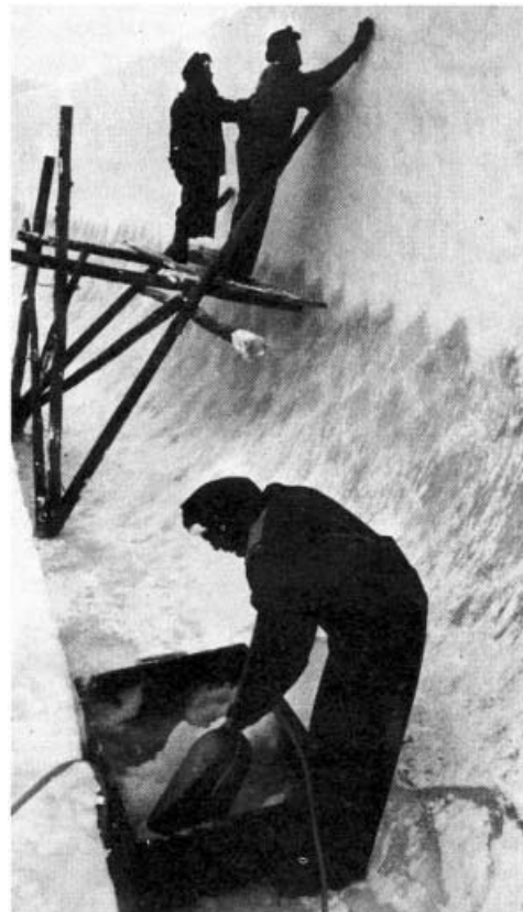
Workers building the bobsleigh course Ouvriers construisant la piste de Bobsleigh
