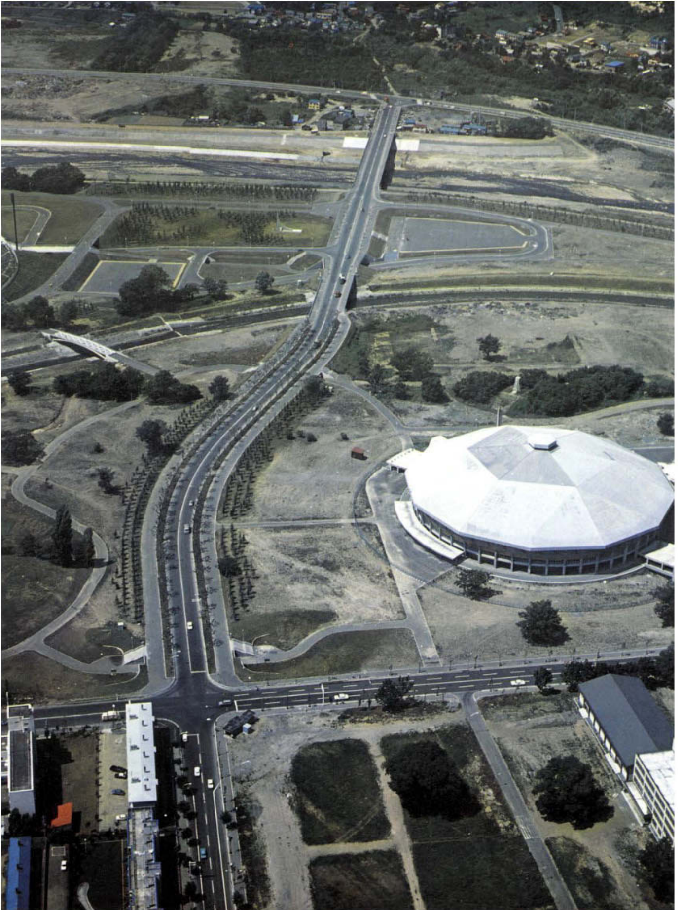
New road linking the site of the Opening Ceremony in Makomanai with the cross-country events site
