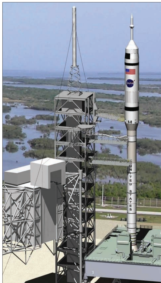
The Ares I-X flight vehicle towers above the shuttle facilities on Pad 39B in April 2009. The pad's shuttle service structures are still in place, and the Ares vehicle uses the shuttle's mobile launch platform.
