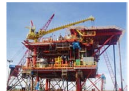
Cashima platform under construction in Trinidad
