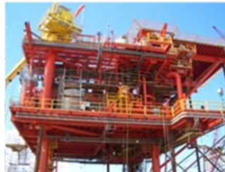
Red Mango platform under construction in Trinidad
