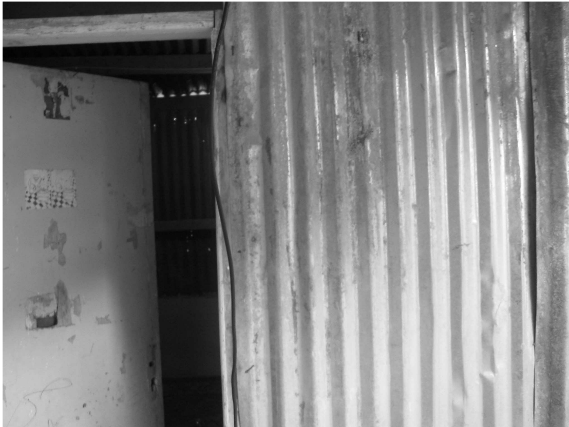
House with corrugated metal sheets in Jal el-Bahr, March 2005, © AI
