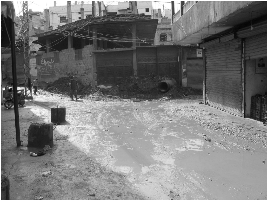
Street flooded with water due to poor drainage system in Nahr al-Bared camp in Tripoli, north Lebanon, March 2005, ©AI
