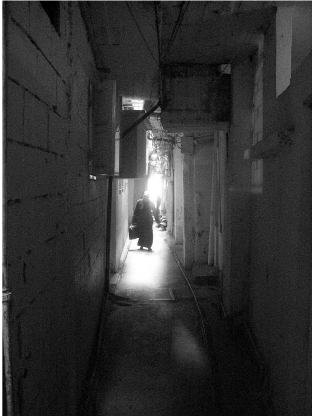
Building extensions blocking out the sunlight in Ein el-Hilweh's alleyways, March 2005, © AI
