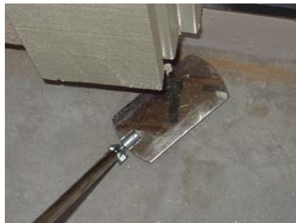
A mirror placed under a door frame reveals a large gap and untreated wood, providing an entry point for insects and water.
