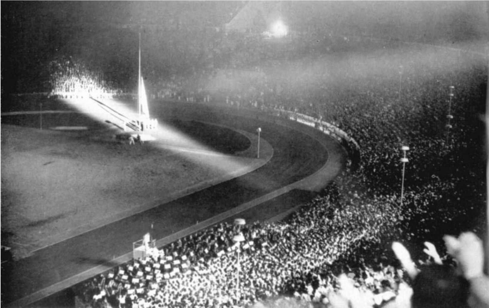
The Olympic Flag is lowered, the Fire dies.
