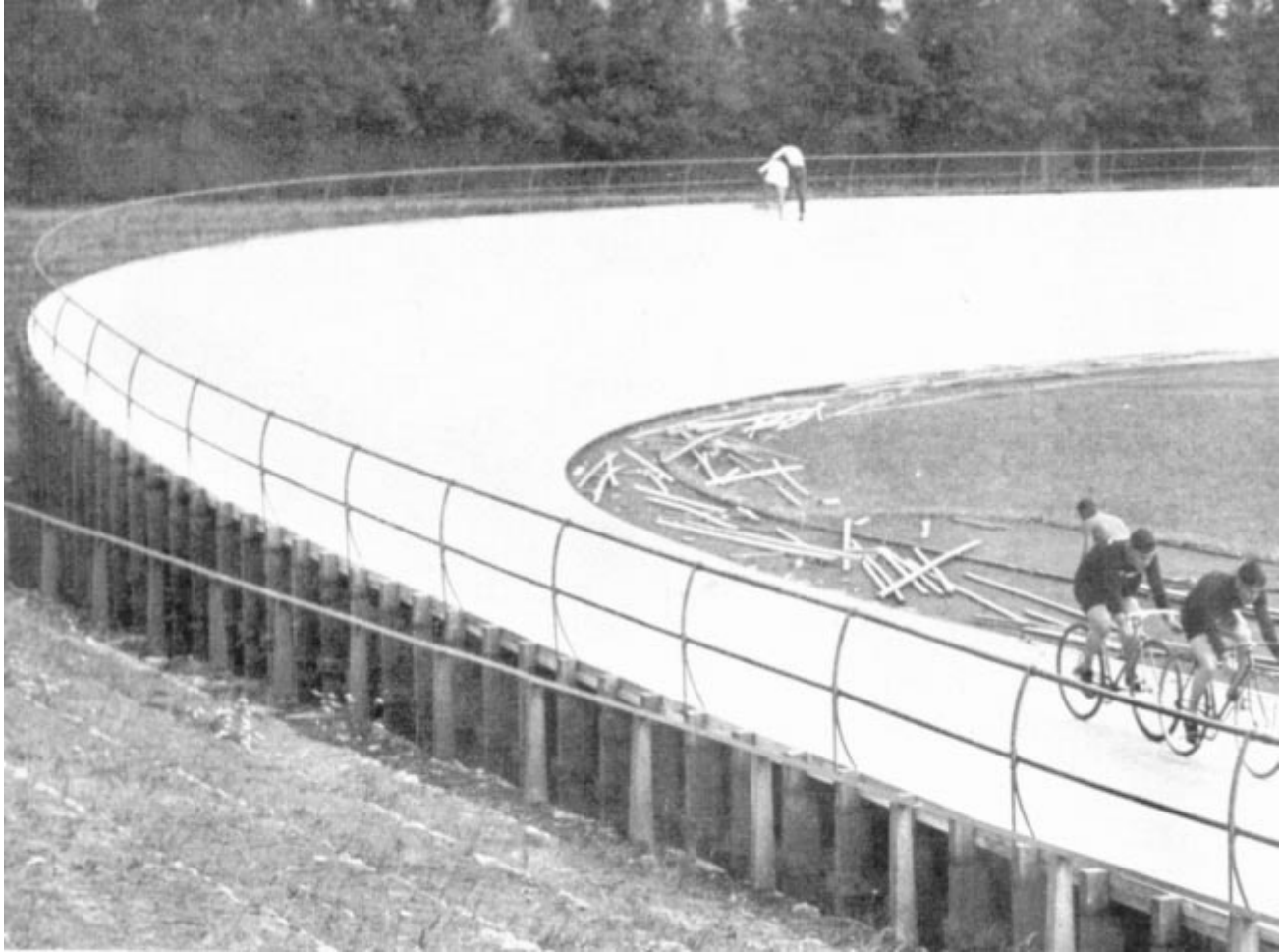
The Australians, Gray and Johnson, training on the newly completed cycling track constructed on a Berlin sport field.
