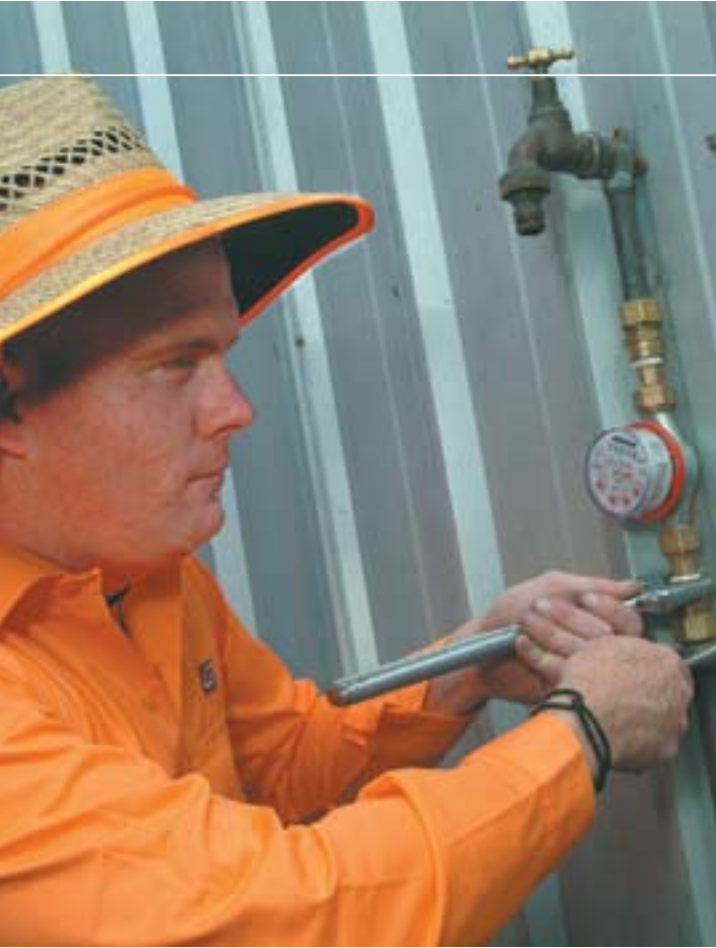
Facilities plumber, Glen, fits a water meter.
