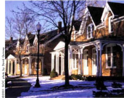
The Olympic Village was located on the scenic University of Utah campus (far left). Center, Olympic Village Director Richard Tyler speaks to the media about facilities as Mitt Romney and J. Bernard Machen observe. The International Zone was in the historic Fort Douglas Officers' Circle, near left.
