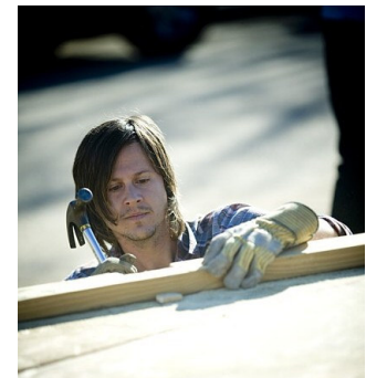
Switchfoot’s Tim Foreman works on a Habitat for Humanity home in Houston.
