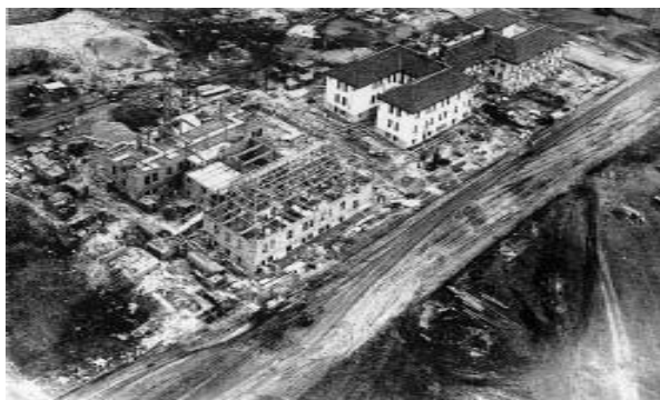
The Bennett Building takes shape
