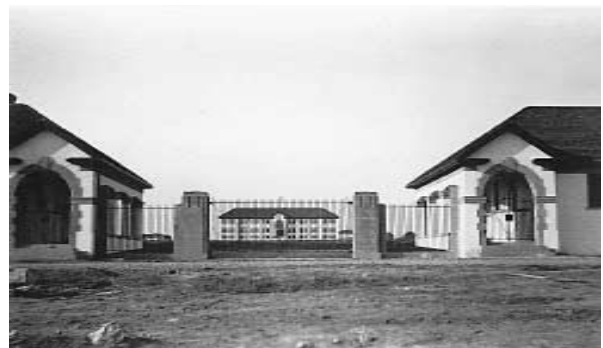
The original gatehouses frame the Athlone Building
