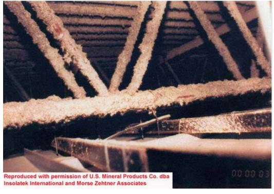
Figure 3-10. Example of damage to SFRM during installation of utilities.
