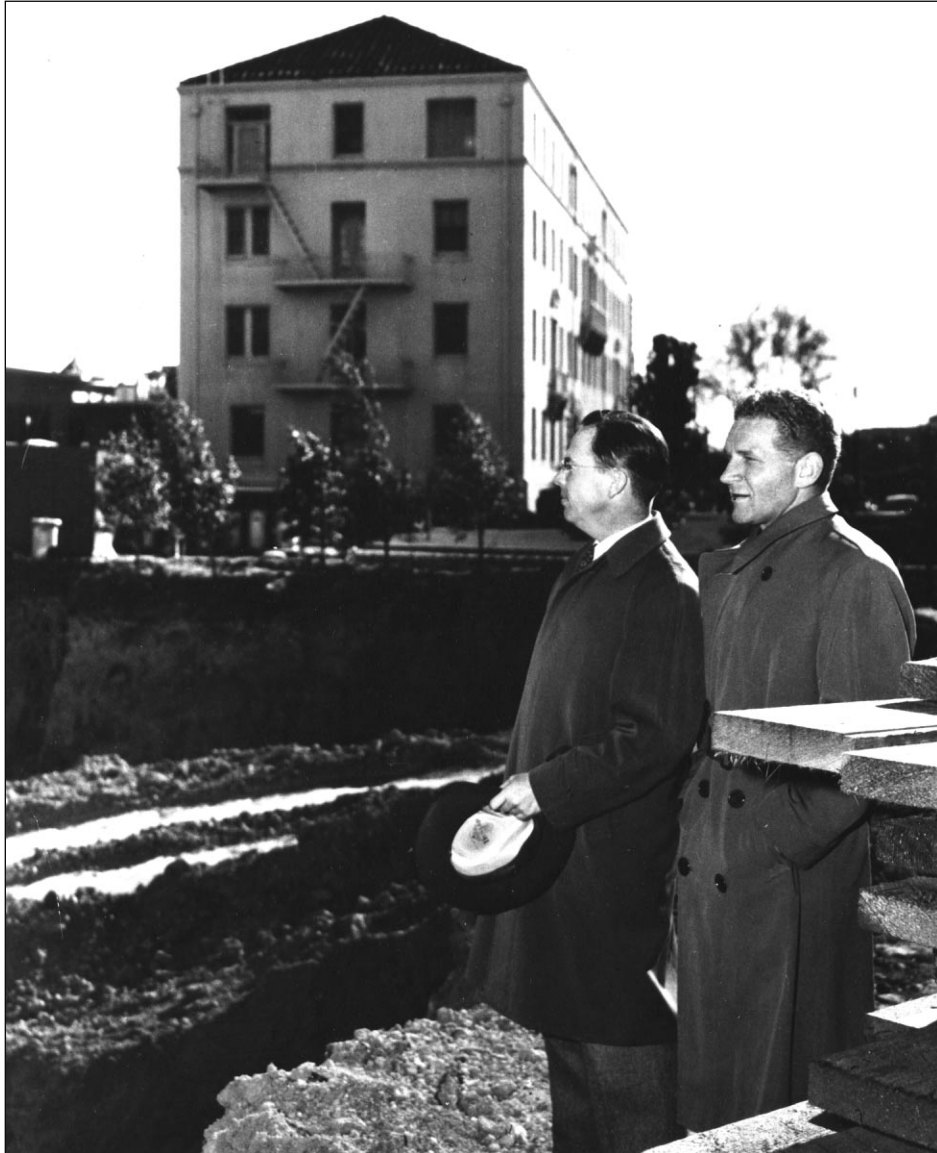
Dr. Garfield, (right) with a Kaiser Company official viewing the building site of the Permanente Foundation Hospital in Oakland, CA, 1942.
