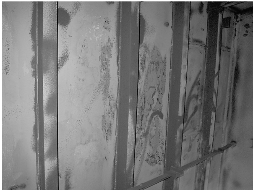
Figure 5.2— Red Beach Bulkhead Stripped of Joinerwork and Water Blasted
