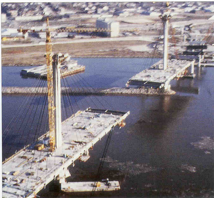
CLARK BRIDGE IS THE FIRST IN THE U.S. IN WHICH SUCH A LIGHT STEEL-FRAMED CABLE-STAYED DESIGN WAS COMBINED WITH A CABLE SADDLE TYPE OF PYLON. THE COMBINATION POSED SOME UNIQUE CONSIDERATIONS FOR CONSTRUCTION ENGINEERING AND ERECTION CONTROL. PHOTO AT LEFT ©1992 DAN SINDELAR.
