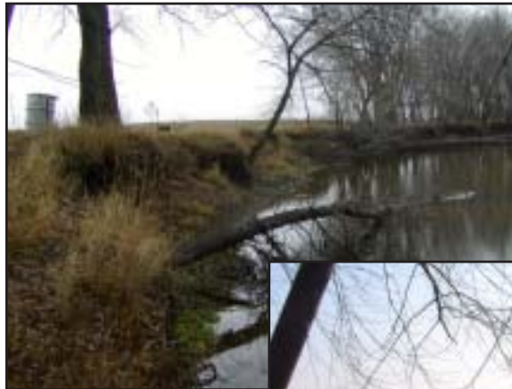
The badly eroded river bank at the Troy Mills Area (left) was armed with riprap (below), protecting the river from sediment and improving fish habitat.
