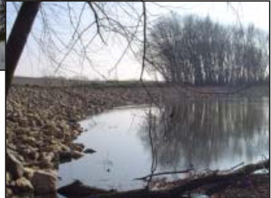
The badly eroded river bank at the Troy Mills Area (left) was armed with riprap (below), protecting the river from sediment and improving fish habitat.
