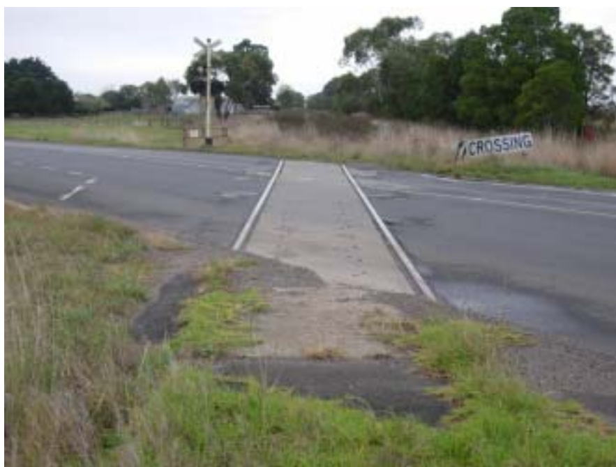
Figure 9-3: Berwick - Cranbourne Road Level Crossing
