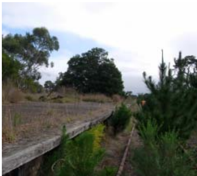
Figure 9-4: Lang Lang Station
