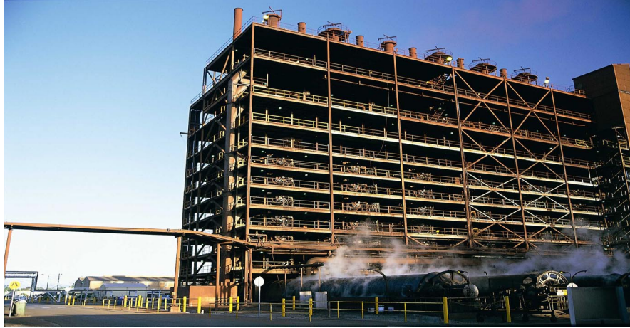
Figure 3. Herreshoff roasters used for reduction of laterite ore
